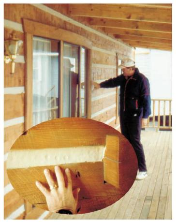
The length of time you'll need to leave the covering in place depends on the weather. If it's warm and dry, the chinking will probably be cured enough in three to four weeks to resist finger poking but if it's cool and damp it may take two to three months before it's safe to remove it. In any case you've probably spent a lot of time, money and effort in obtaining a great looking chinking job and protecting it for a few weeks is well worth it.
