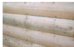
Dark colored streaks from metallic tannates. Oxcon solution will remove rust stains caused by nails, screws and fasteners.
