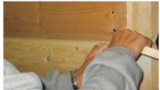
Installing masking tape backing.
