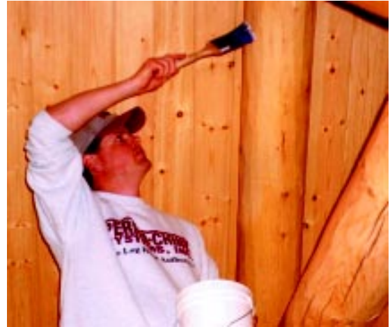
Application of Acrylic Gloss finish on interior log wall
