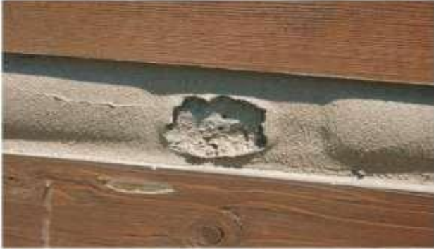
Blister Formed by Entrapped Air or If Chinking Was Applied in Hot Sunlight.
