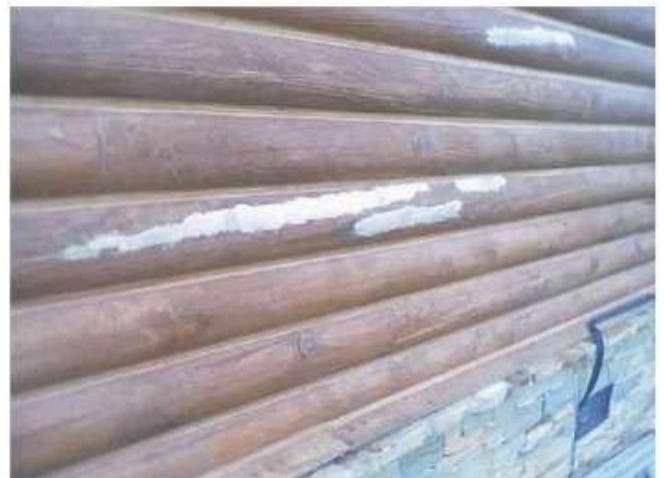
Voids treated with Shell-Guard RTU, M-Balm then filled with 2x4s and E-Wood.
