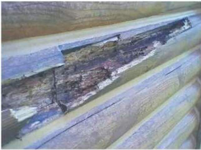
Large voids in logs after removing soft, loose wood fibers.
