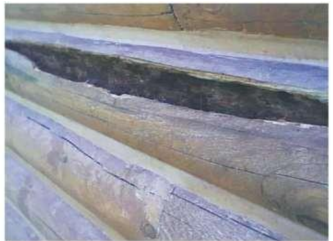
Large voids in logs after removing soft, loose wood fibers.
