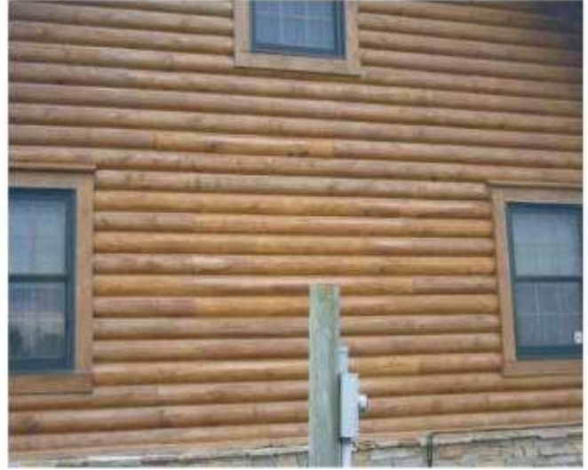
Repaired areas coated with Energy Seal then stained.
