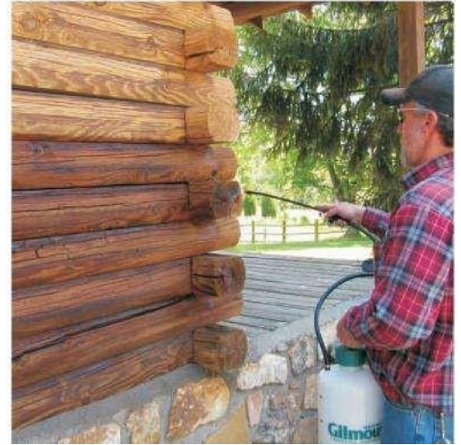
Applying a borate solution
