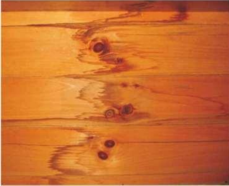
Interior Water Stains Under a Finish
