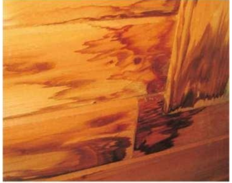
Interior Water Stains Under a Finish
