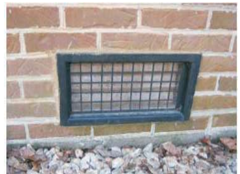
Sealing foundation vents
