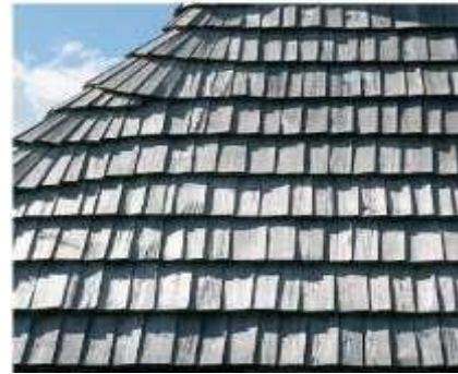
Weathered Shake Siding
