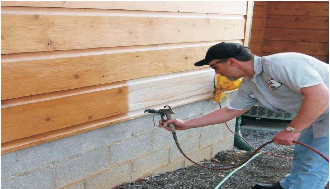
Applying S-100 Finish Remover Using a Wagner 9140S Airless Sprayer
