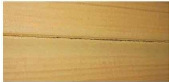
Split along siding seam.
