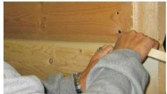
Split along siding seam.
