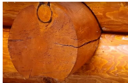
Cured Log End Seal
