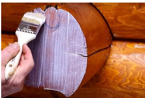
Application of Log End Seal
